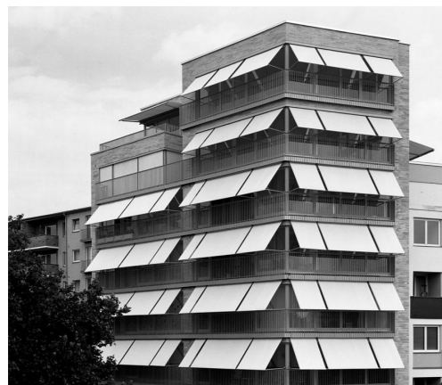
Apartmenthaus Kurfurstendamm. Heide von Beckerath Alberts. Berlin, Alemania (2000-2006)
